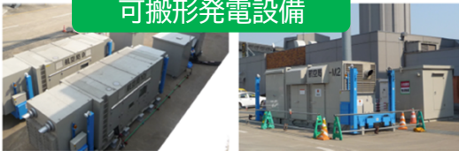
Secondary Power Supply
